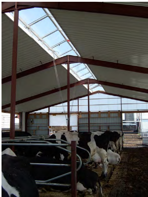
Arntjen ISO lighting/ventilation ridge on top of a shed in the USA
